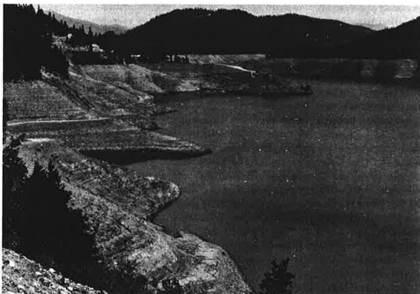
California drought. Researchers in the San Francisco Bay Area are studying supplier and consumer reactions to the 1977 water shortages with the objective of recommending better water management strategies. The impact of that drought is seen in two views of Clair Engle Reservoir, full (2.4 million acre-feet) in 1974 (left page) and down to 460,000 acre-feet in August 1977 (above). (Photos by U.S. Bureau of Reclamation)
