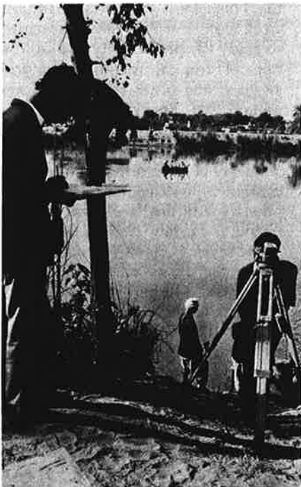
Water research. As part of a U.S.-Pakistan joint research project, scientists (left) meter the water surface level of a Link Canal and take a soil core (right) to determine particle size of bottom sediments. The Link Canals, built to redistribute scarce water among Pakistan's rivers, are part of one of the world's most ambitious water development projects. Their size and variety make them valuable for research on the design of modern irrigation channels. (Photos by Kahlid Mahmood/George Washington University.)
