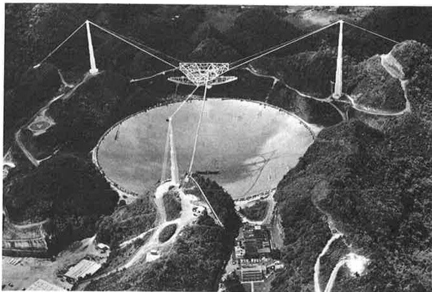
The National Astronomy and Ionosphere Center's upgraded radio-radar telescope near Arecibo, P.R., has a newly panelled surface and upgraded electronics that increase its planetary ranging and mapping capability a thousandfold. [Photo by Cornell University]
