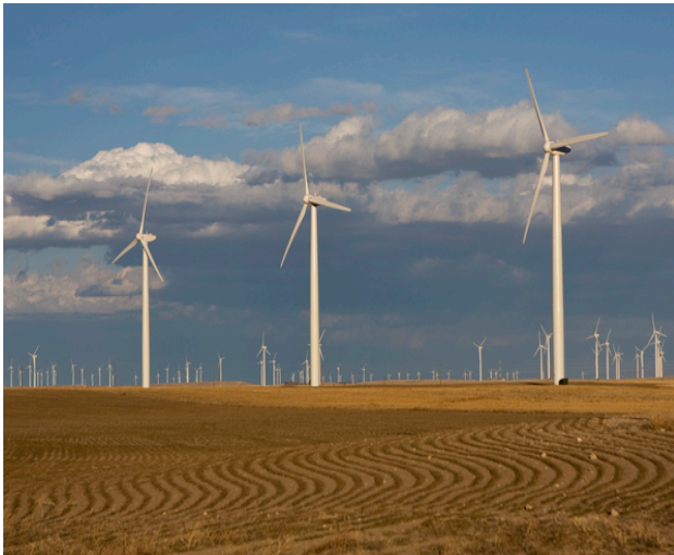
This image shows turbines on the Cedar Creek wind farm with plowed fields beneath.
